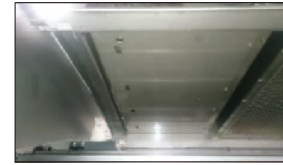
刚完成清洁时 After cleaning
